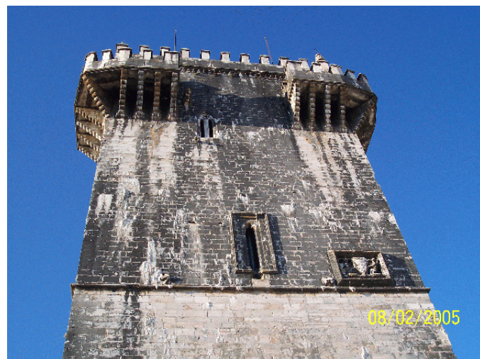
Looking up to the tower.
